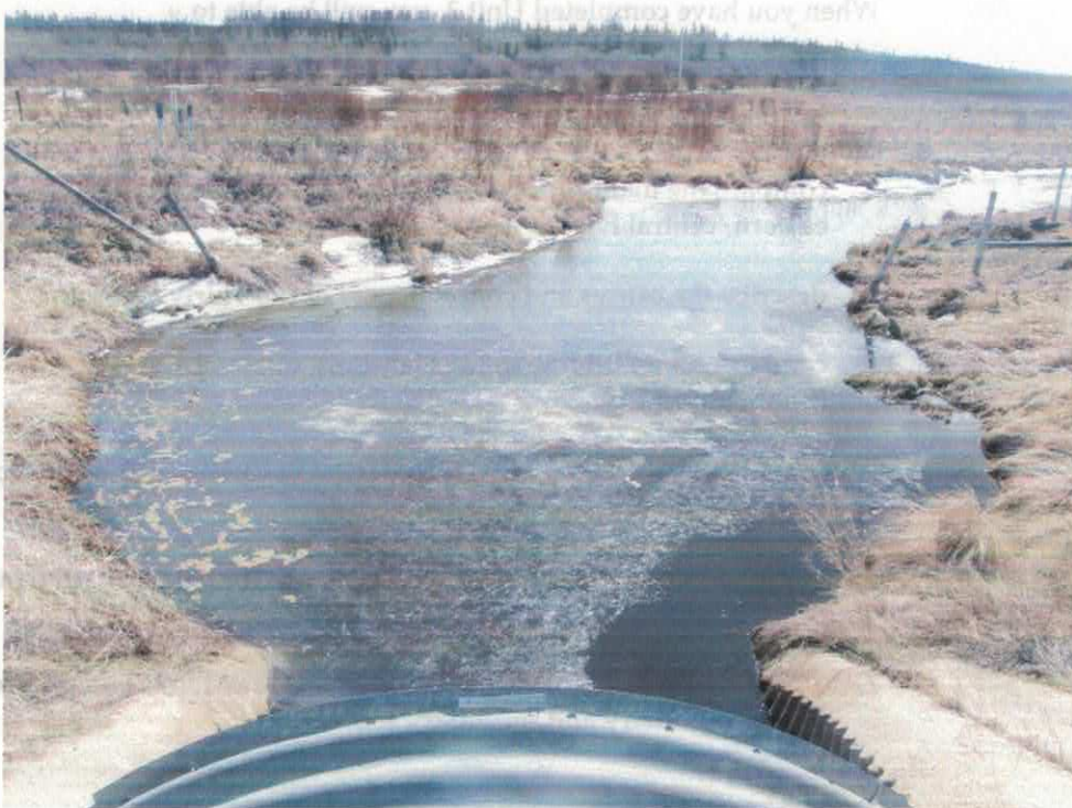
Photo # 14. Looking N over large culvert at streambed where cattle have direct access and there is little riparian veg left and evidence of nutrient enrichment by presence of Lemnna duck-weed at location TW06 NW of Tawatinaw on April 21, 2011
