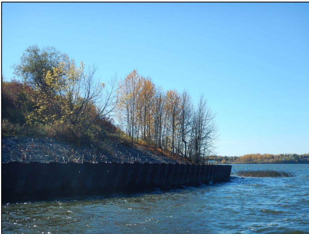
Photograph 9. Retaining wall located near Lac La Biche in shoreline segment 1.
