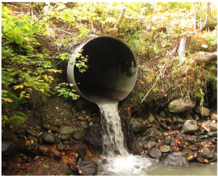
The mouth of this culvert has eroded over time and is no longer allowing fish to move upstream. Culverts that are too narrow or too wide can change stream properties, particularly flow velocity but also water depth and temperature.
